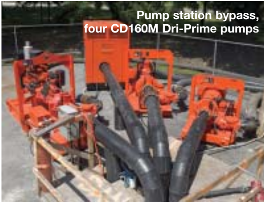
CD150M Hush-Pac 150mm Dri-Prime for Stormwater Sewer Bypass
