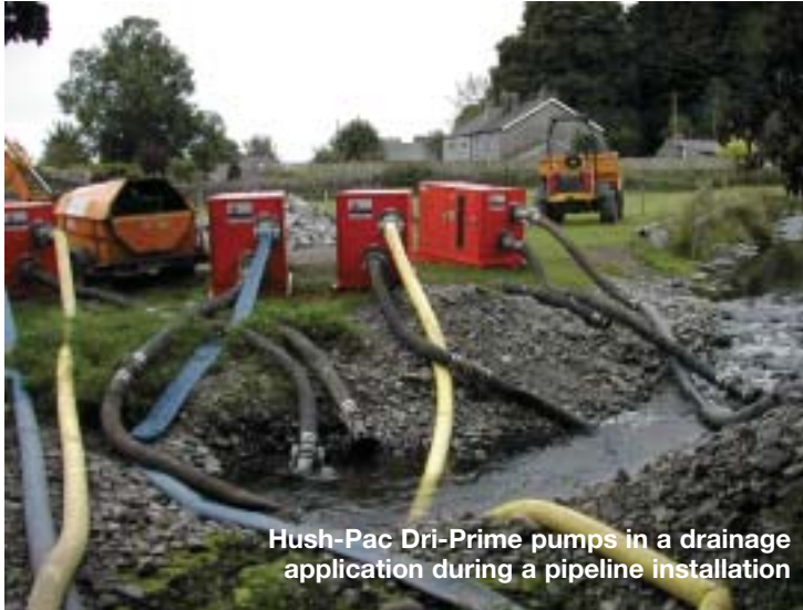
136,000 M 3 /day bypass, seven 300mm pumps, 5 month duration
